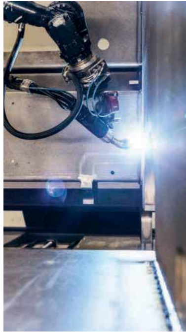
LaserHybrid welding is a combination of two different welding processes: laser welding and Gas Metal Arc Welding (GMAW)
