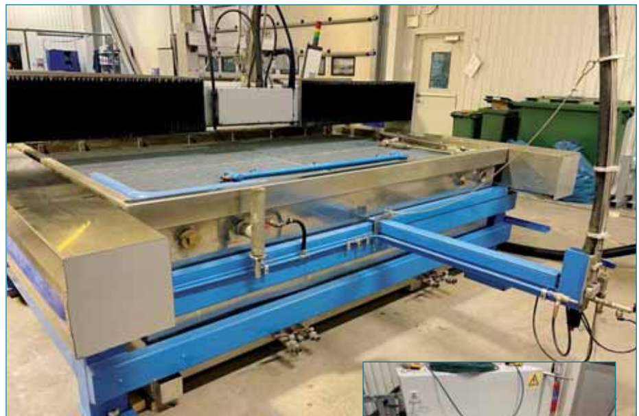
The machine is completely renovated, on all sides and equipped with new cables and a new operator panel
